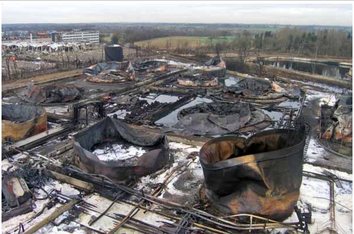
Figure 3.2 Devastated tanks after the fires © the Hertfordshire Fire and Rescue Service
