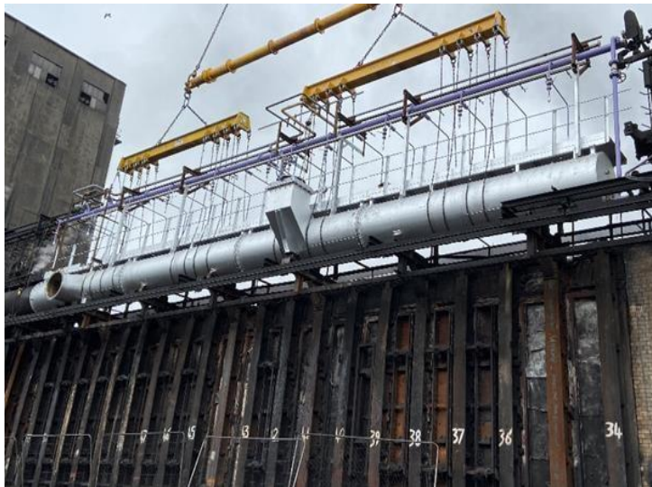
Figure 3. New Battery 2 gas collector main being lowered in to position
