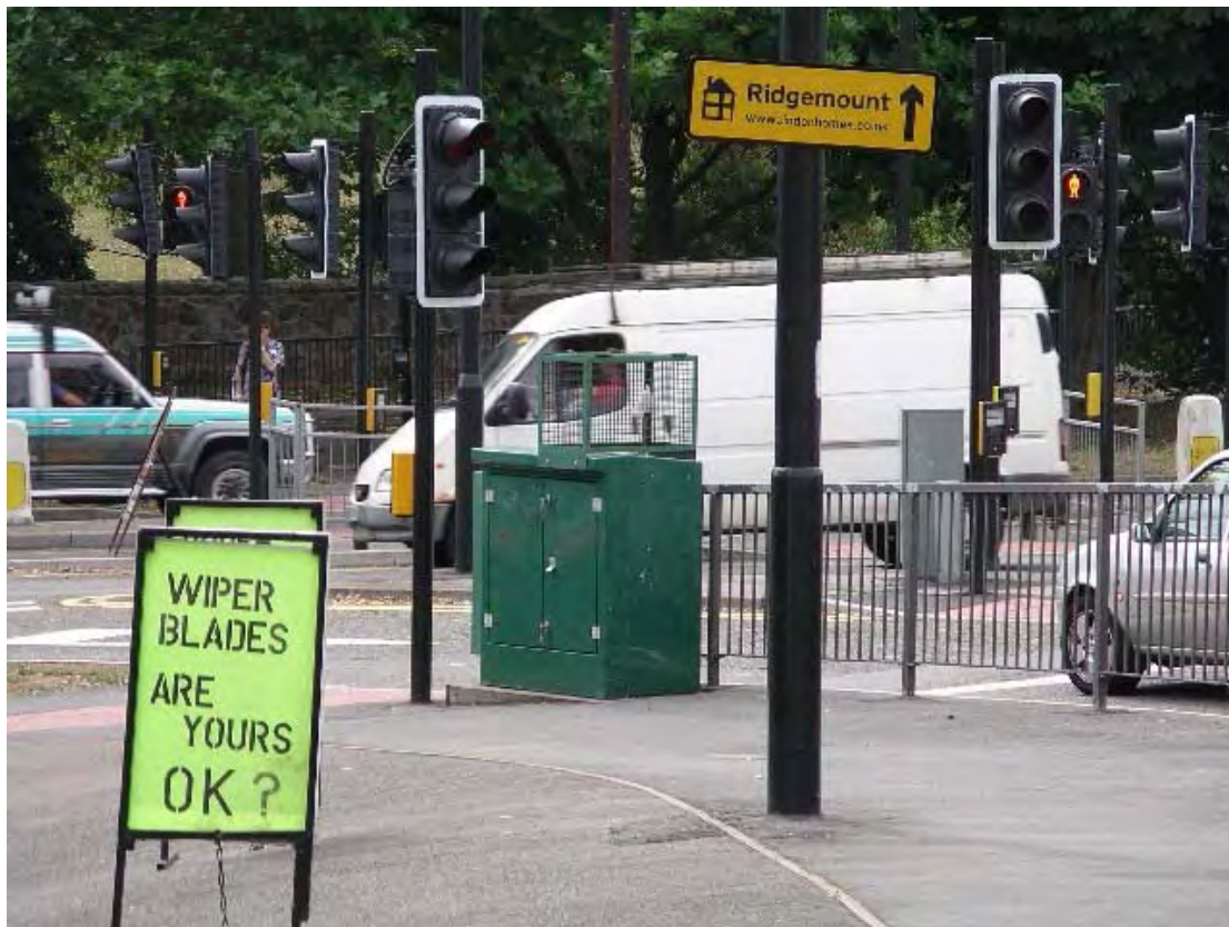
Figure 27 Photograph of location of Wells Road NO x analyser
