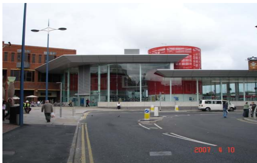
Figure D3: The new Bus Station.
