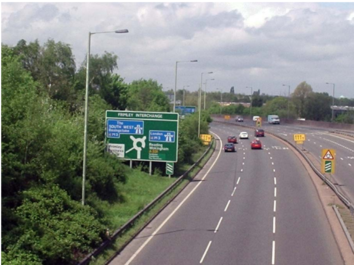
Photo 2: A331 approach to J4 of M3
