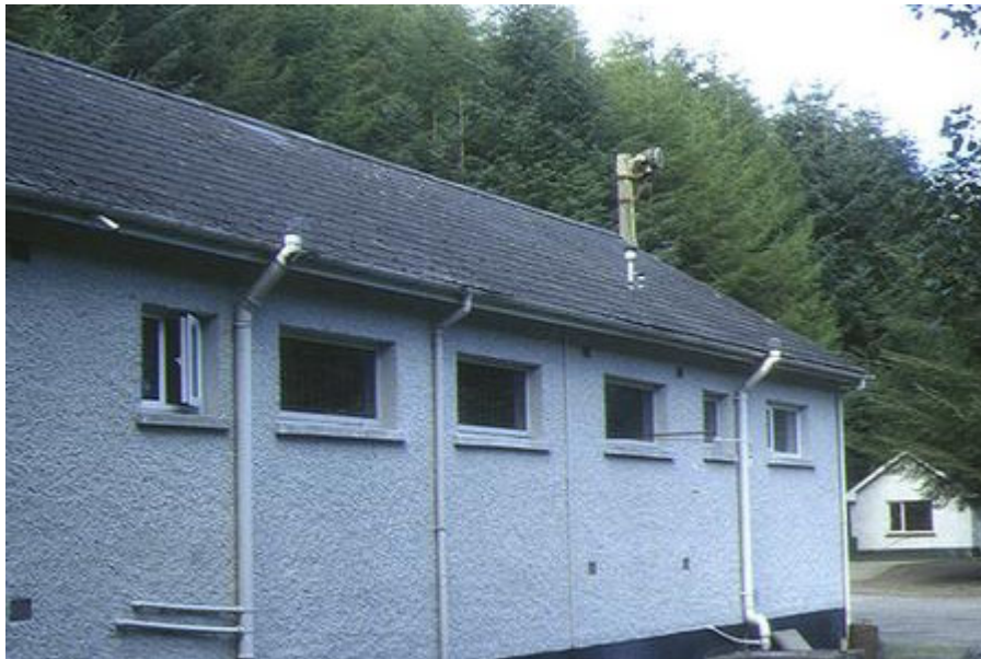
Figure 7.2 Lough Navar AURN Rural Site (analyser is inside building).
