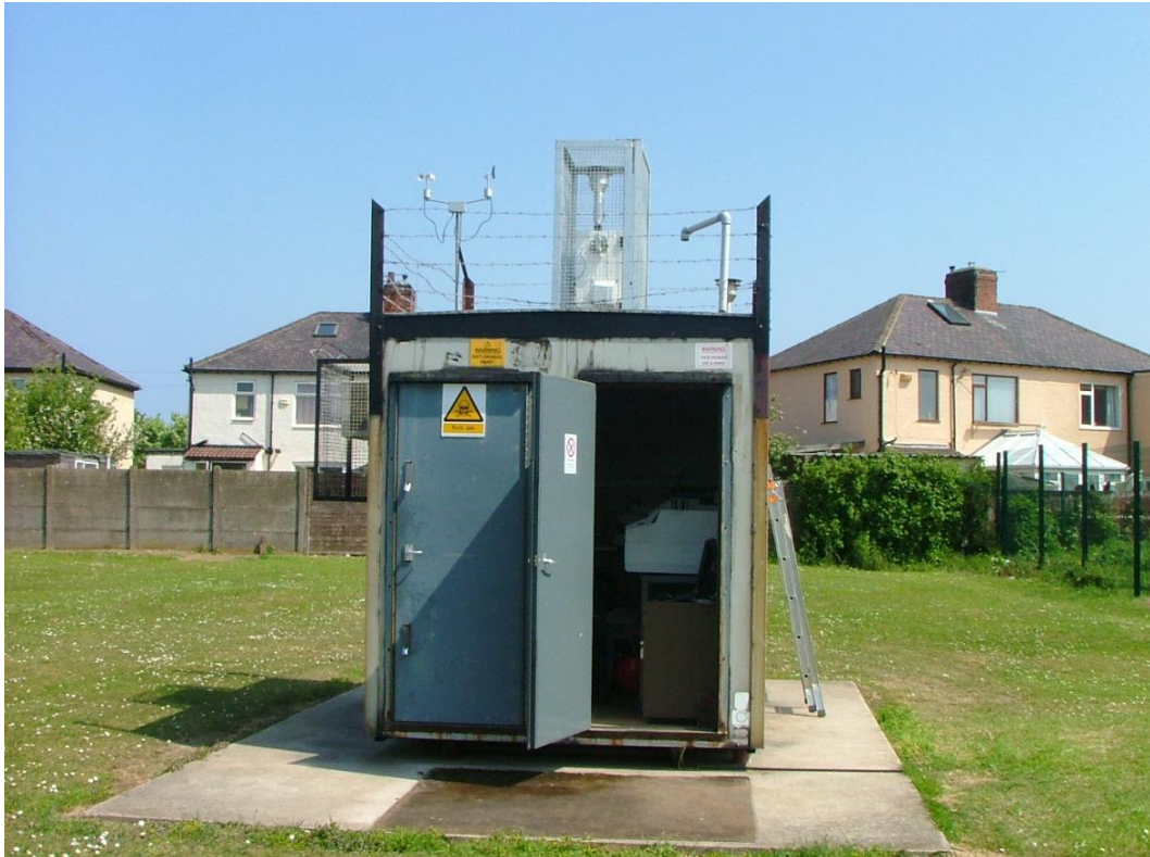
Image 1. A site audit in progress at the Redcar AURN Network site in May 2008. The Partisol 2000 sampler is visible in the cage on the top of the monitoring cabin.
